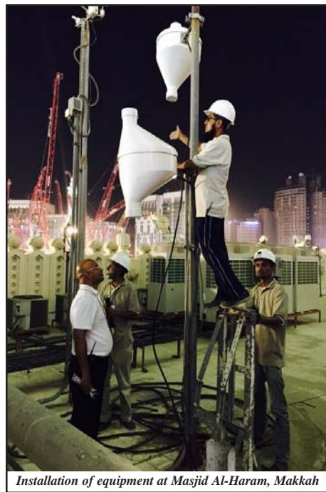
Installation of equipment at Masjid Al-Haram, Makkah
