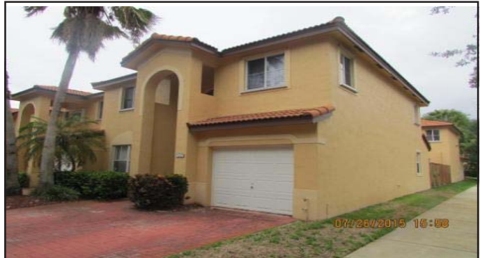
House in Davie, Florida USA
